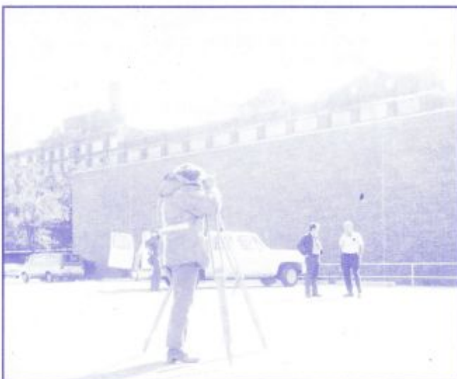
Surveying for Building 36 addition, October, 1974.
