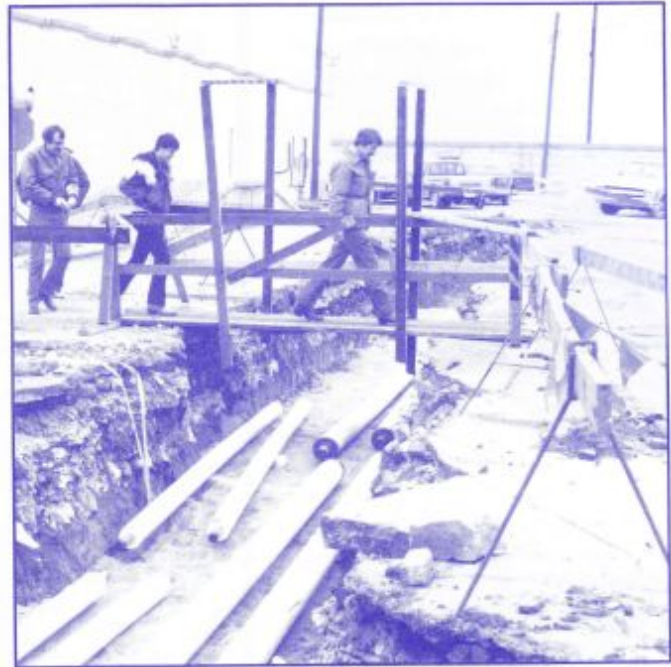
March, 1986: Employees leaving the Dining Hall cross a "moat" necessitated by installation of a heating/air conditioning loop to serve the outlying buildings at 3200 S. 2nd St.
