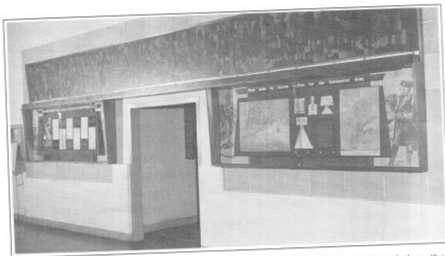
Limestone lithographic stones border the exhibit cases and wall mural displayed along the north wall of the Erskine Hall lobby area in 1963. The stones were eventually covered with layers of paint and spackling. Current construction efforts have led to the lithostones' discovery. Photo provided by Tom Yanosky.
