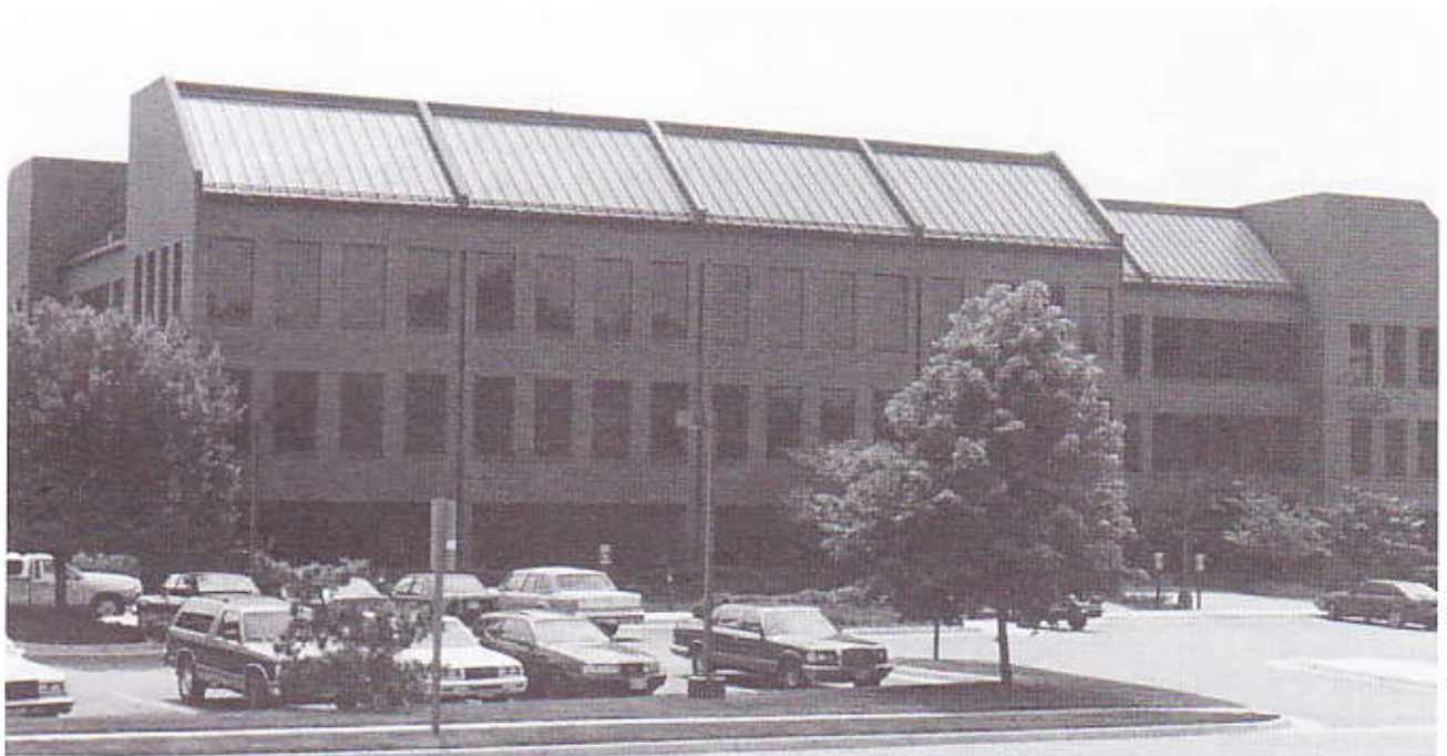
Central Imagery Office headquarters building
