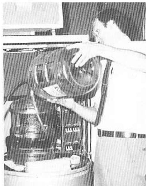
COOL IT —A contractor pours a bottle of distilled water into the cooling system of the Sperry 1100/91 computer system, installed in the Geosciences Division at South Annex. The top-of-the-line system, described as a "numbers cruncher" because of its computational power, was the first of three 1100/91's to arrive at the Center as part of the modernization program. (Photo by John LaBuster)
