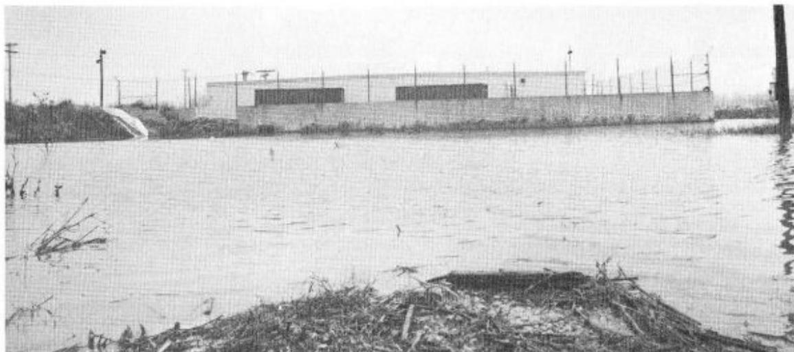
River Des Peres, which normally flows to the north (right) of Building 4, laps the eastern side of the floodwall protecting the building. The large hose running down the bank at left was used to discharge runoff that normally empties from a pipe leading under the building. During the flood of 1973, hundreds of employees volunteered their labor in a massive sandbagging effort at South Annex. The floodwall was constructed soon after. (Photo by John LaBusier)
