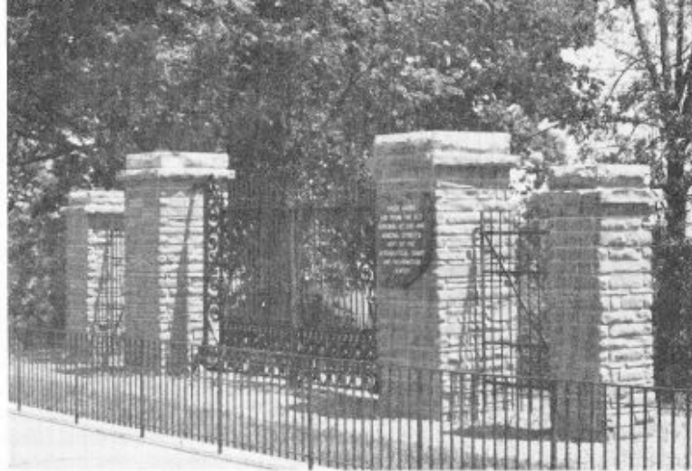
This was the main land gate of the St. Louis Arsenal. Built about 1845 it was originally located in the installation's north wall. Later it was moved to the position of the reservation's present main gate. Later still, it was taken down and stored. In 1952 it was given to St. Louis County's Jefferson Barracks Historical Park where it was reerected and is now on public view as shown here.
