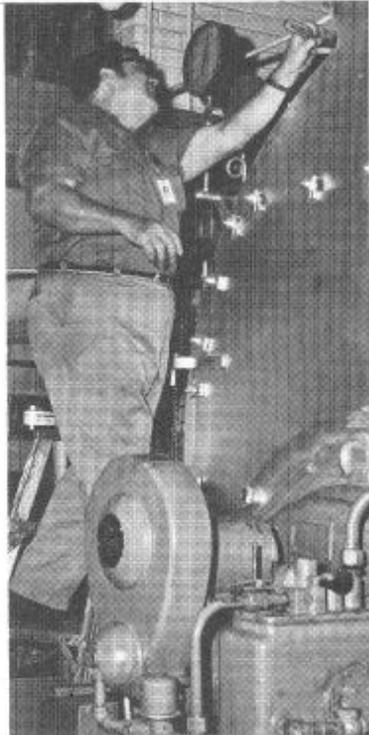
Bill McNichols adjusts quadrant damper for greater boiler efficiency.
